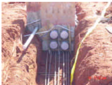
Ductbank – once built invisible
